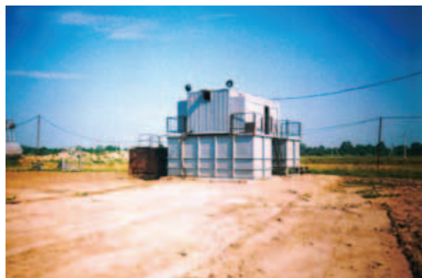
Figure 2.132. Installation of ECHO-B-3 to treat drilling wastewater from regional LUKOIL enterprises.
