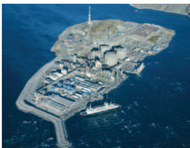
Figure 2.138. The Melkøya LNG plant and terminal.
