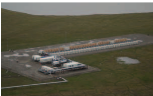
Figure 2.129. Recent Development Gravel Pad with 10-15 foot well spacing.
