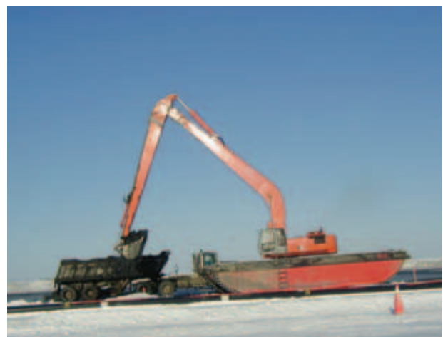
Figure 2.39. Northstar pipeline trenching operation (MMS).
