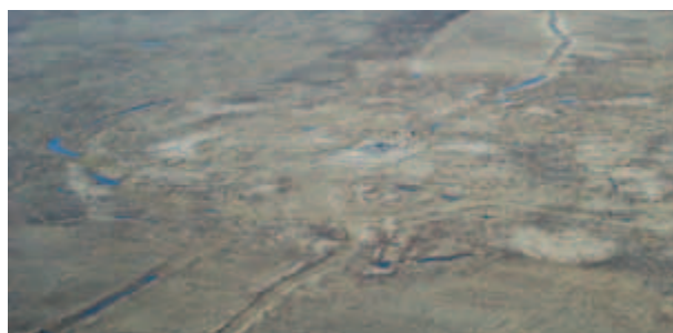
Figure 2.118. Above: Fish Creek No. 1 well site in 1949. Bottom: Tundra scarred by tracked vehicles and the concrete cellar for Fish Creek No. 1 well today.
