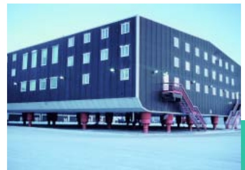
BP operations center, Prudhoe Bay, Alaska, built on pilings to resist damage from thawing permafrost.
