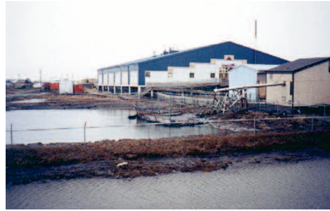
Fig. 15.17. Lagoon waste washed through fence by storm surge flooding, Kipnuk, Alaska (photo by Brian Aklin).
