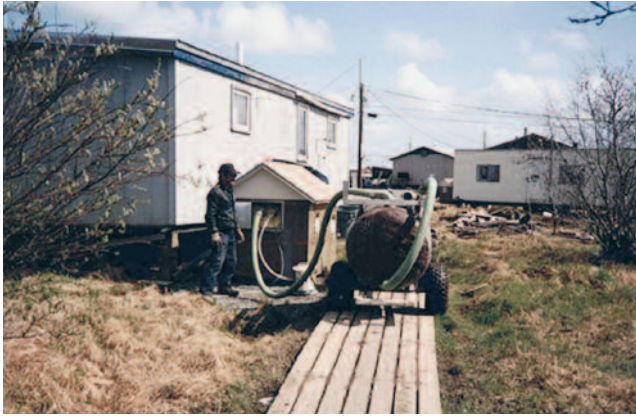
Fig. 15.16. Small sewage haul system, Mekoryuk, Alaska (photo by Mark Baron).
