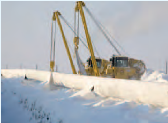
Figure 10.5. Pipeline under construction in the Russian Arctic.
