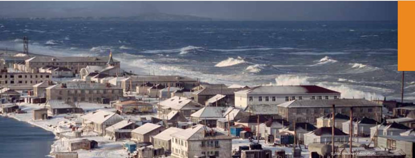
Less sea ice in recent years has resulted in more storm damage to buildings in the coastal settlement of Uelen, Chukotka, Russia.
