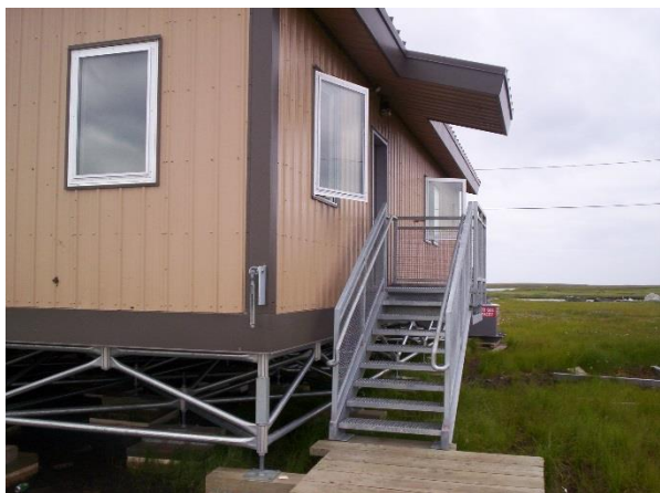
A multipoint structural foundation used to maintain stability of buildings on thawing permafrost, Newtok, Alaska. Credit: Alaska Department of Military and Veterans' Affairs
