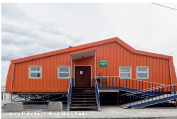
Health clinic, Yanrakynnot village, Chukotka
