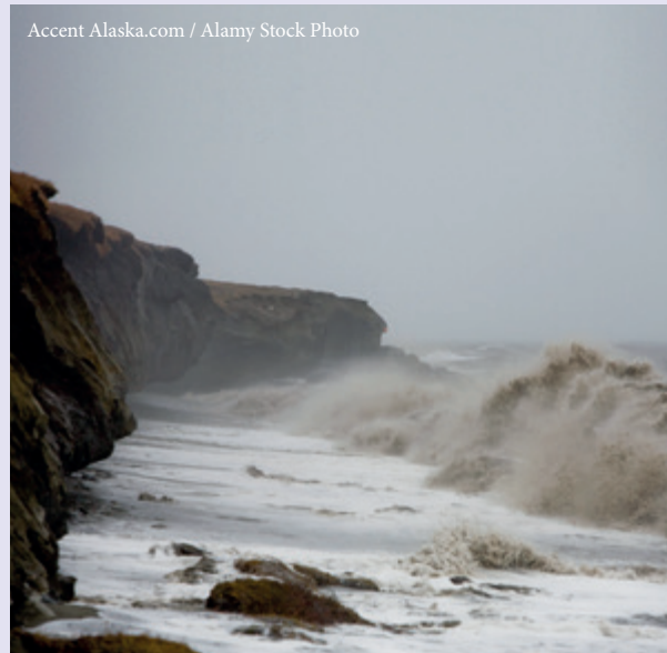
Erosion of coastal permafrost during a winter storm
