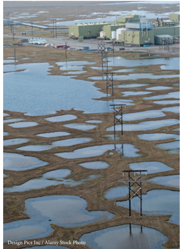
Aerial view of electric transmission lines over tundra leading to an oil development structure in Prudhoe Bay, Alaska
