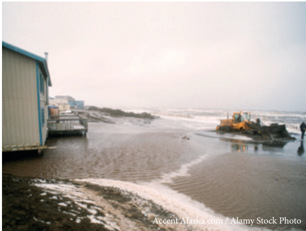
Bulldozer on beach attempting to build levees against an approaching storm, Utqiagvik, Alaska
