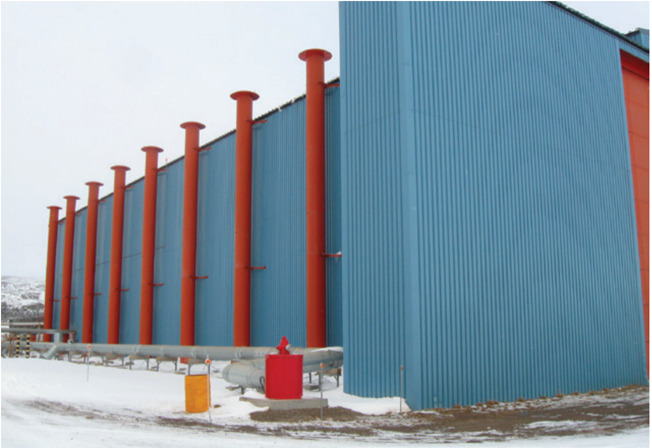
Figure 10.18 Aircraft hangar under-floor cooling plenums, Thule Air Base (photo by Kevin Bjella).
