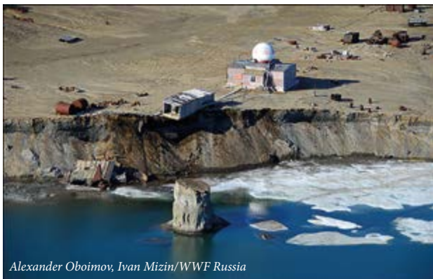
Figure 2.8 Coastline erosion is observed at some locations to exceed 30 m/y, and is 5 m/y on average. The image shows an abandoned meteorological station on Vise (Wiese) Island falling into the Kara Sea (Gertcyk, 2016).
